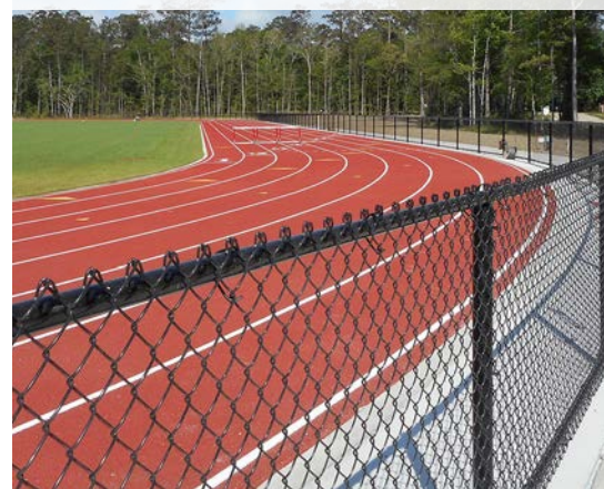
VINYL-COATED CHAIN LINK FENCE (6')
